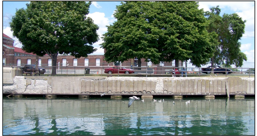
LaSalle seawall protecting the Colonel F.G. Ward Pumping Station.
